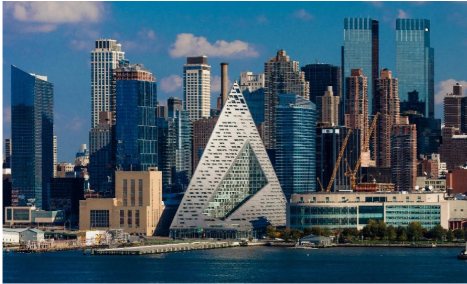
Via 57 West in New York City: This ultra-modern, innovative residential complex was built using structural concrete block, cast-in-place concrete flooring, and precast concrete stairs made with ground-glass pozzolan to help meet sustainability goals.
