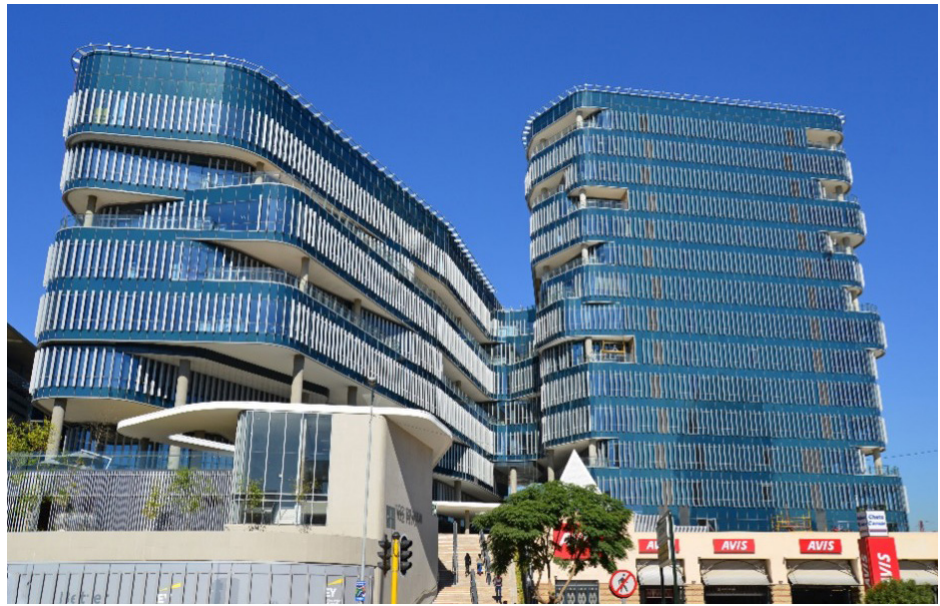
102 Rivonia in Johannesburg, South Africa, used fly ash in the concrete to reduce the overall cement use of the project by 30 percent, which heavily contributed to the project having a lower carbon footprint.
