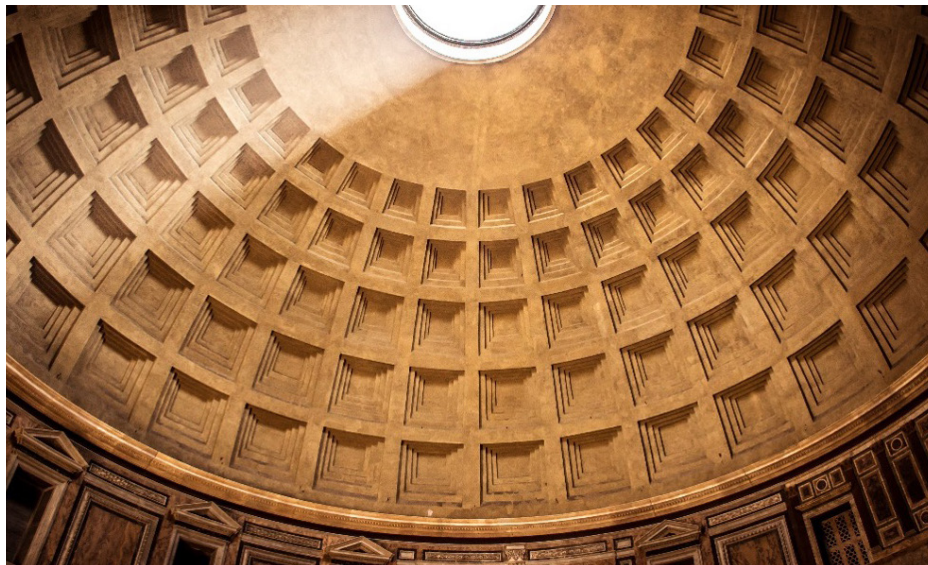
The Romans built the Pantheon—which is still the largest unreinforced concrete dome on earth—with hydraulic cement made from natural pozzolans.
