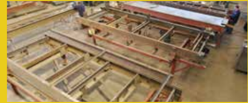
Raw steel is fabricated.
