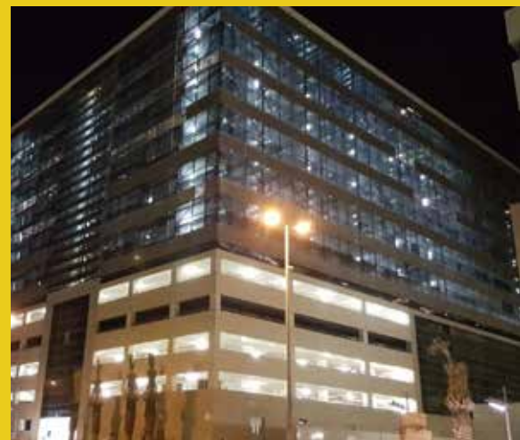
The building facade is independent of the parking garage. In this case, the APS is installed above a conventional parking garage.
