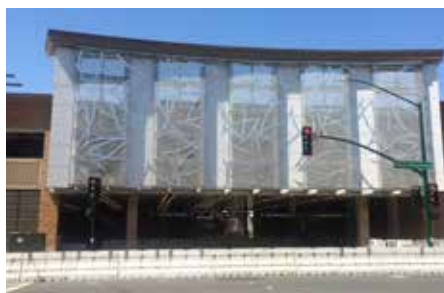
Exterior facades can be created with coiled wire fabric that offers an appealing design by day and a dynamic lighting option at night.
