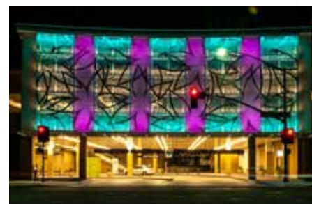
Exterior facades can be created with coiled wire fabric that offers an appealing design by day and a dynamic lighting option at night.
