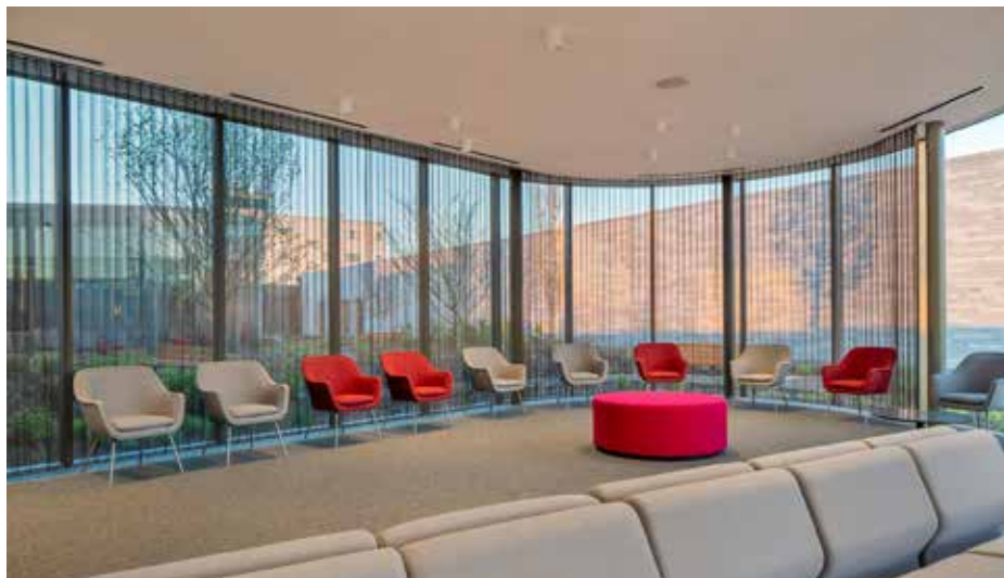
Coiled wire fabric can be used on interiors as a durable, appealing, window treatment to control glare but still allow for daylight, views, and HVAC operation at the windows.
