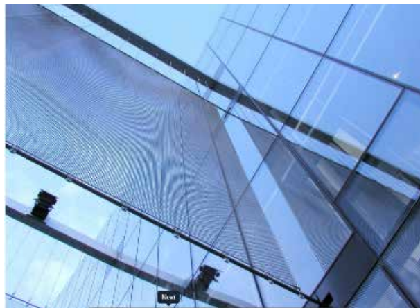
Attachment systems for coiled wire fabric are typically based on frames or tracks that can be designed to suit different shapes, sizes, and installations.
