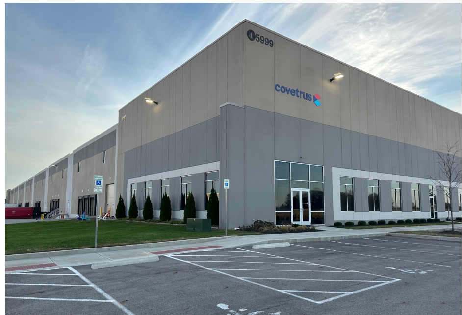
This building was built with precast, or tilt-up, construction, which requires a two-step installation process: large concrete panels are cast on site, which are placed in position by a crane.
