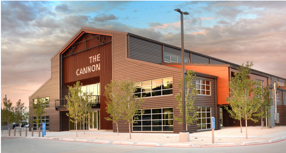
The Cannon, an entrepreneurial hub in Houston, Texas, called for more than 90,000 square feet of insulated metal panels (IMPs) for walls and roofing.
