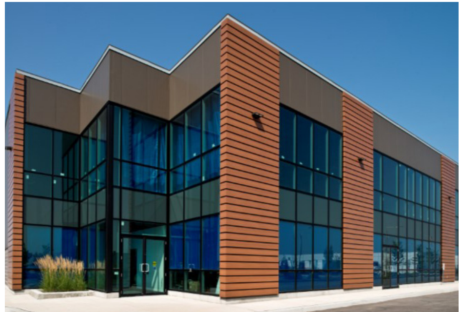
This multi-tenant, mixed-use building on a prominent corner in Vaughan, Ontario, features insulated metal panels in dark bronze which complement the wooden panels.
