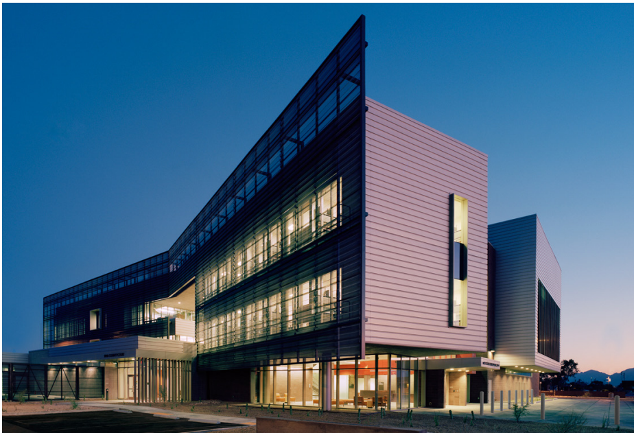
Designers of the University of Arizona Medical Center South Campus building in Tucson, Arizona, chose IMPs to meet short construction deadlines, high design standards, and demanding environmental conditions.
