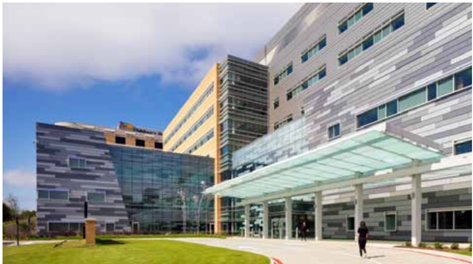
Metal composite material (MCM) is a popular aesthetic choice for architects. It is cost-effective and, being made of 70% recycled material, meets sustainability goals.
