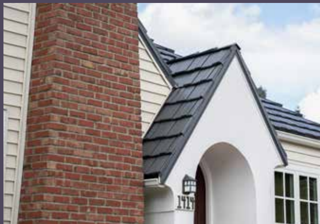
A home located in Seattle was renovated with weather-resistant metal shake roofing.
