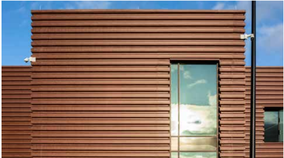
IMP walls come in a variety of colors to match any aesthetic, such as the earthen, prairie color in this close up of the Williston Basin International Airport.
