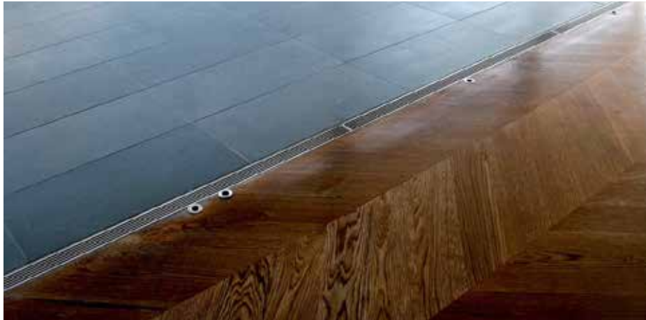
Decks and patios covered with tile or solid, continuous surfaces benefit from the design integration of architectural linear drains.
