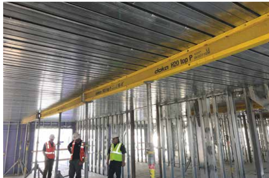
Long-span composite floor systems can reduce weight, interior supports, and overall project time and costs.
