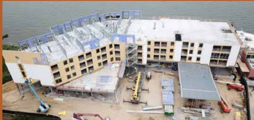
Photos: Richard Jarvis, courtesy of New Millennium Building Systems
