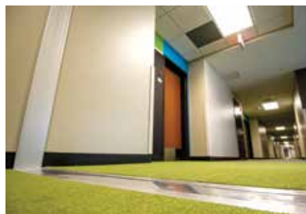
The form and appearance of expansion joints in multifamily buildings can vary based on the selection of type and materials.
