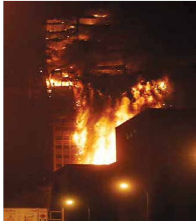
This photo of the Windsor Tower located in Madrid, Spain shows the results of “leapfrog” fire propagation. Note how the fire has spread vertically along the outside of the high-rise.
