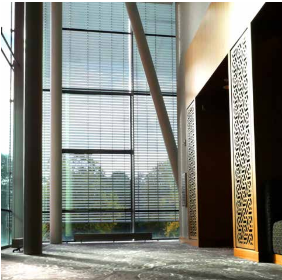
Exterior shading systems like these venetian blinds maximize ambient light entering the building while preventing direct sun penetration.
