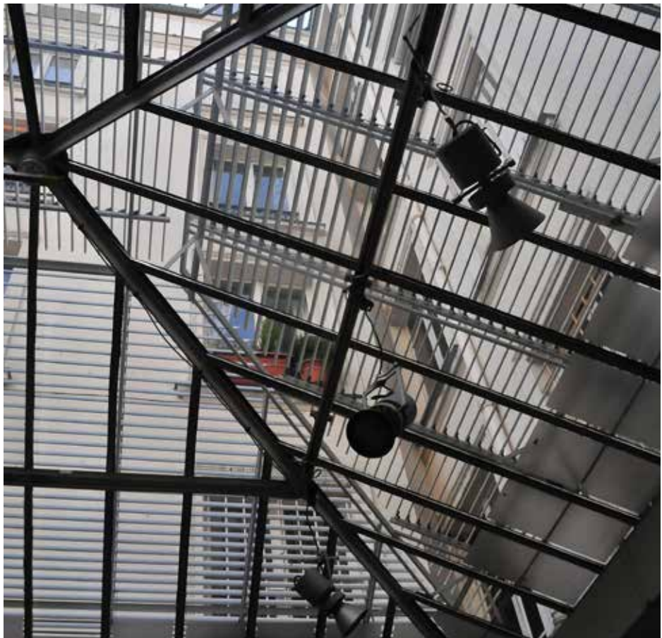
Rack arm shading systems offer a high level of versatility and can therefore match any type of shape or glazing orientation.
