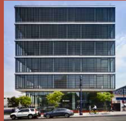
BNIM's LEED Platinum net-zero design for Makers Quarter Block D in San Diego features an exterior venetian blind system linked to an automated sun-tracking system so that it is automatically deployed and tilted to prevent direct sun penetration.
