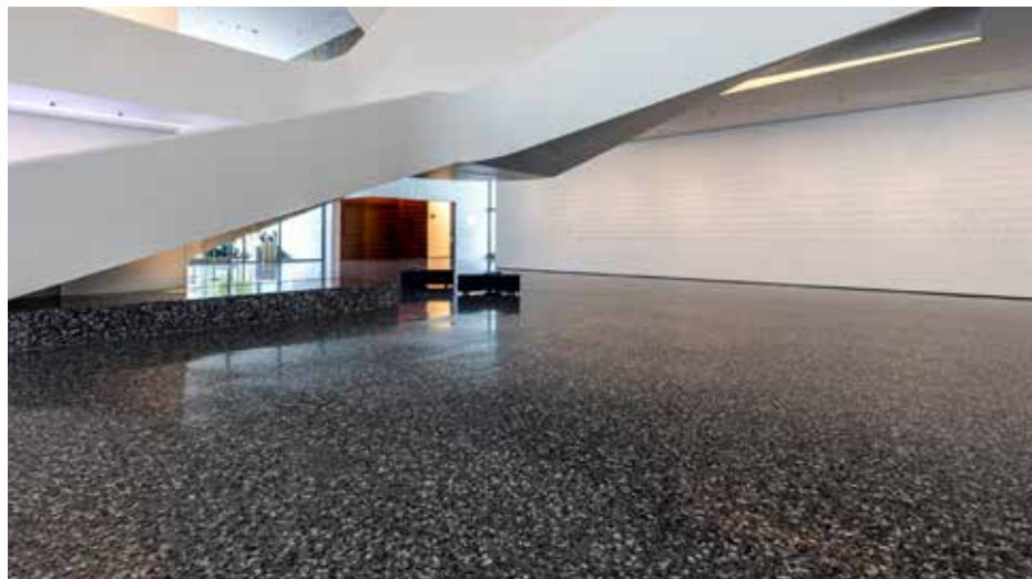
At Houston's Museum of Fine Arts, terrazzo is significantly featured in flooring, staircases, raised seating, coves, and a plinth.
