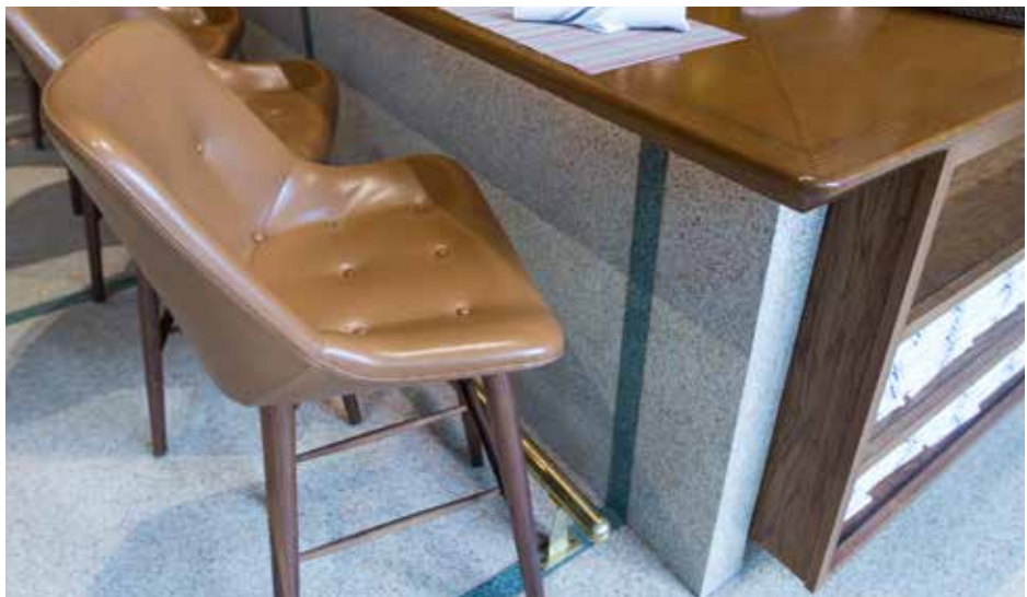
A terrazzo bar front and floor-to-ceiling terrazzo surfaces deliver a beautiful aesthetic for the adaptive reuse of a mid-century bank building into the boutique Fairlane Hotel in Nashville.
