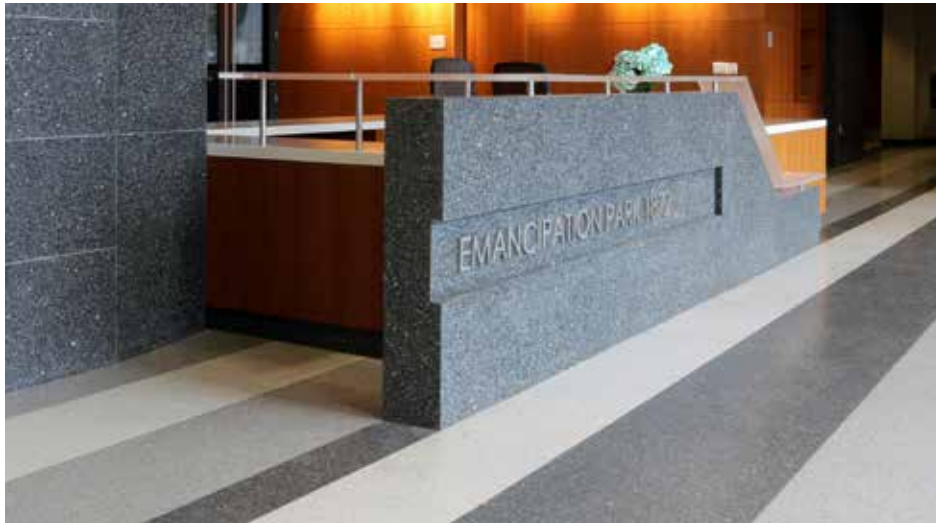
White and gray precast epoxy terrazzo was designed for the desks, walls, base, and donor wall at Emancipation Park Community Center in Houston.
