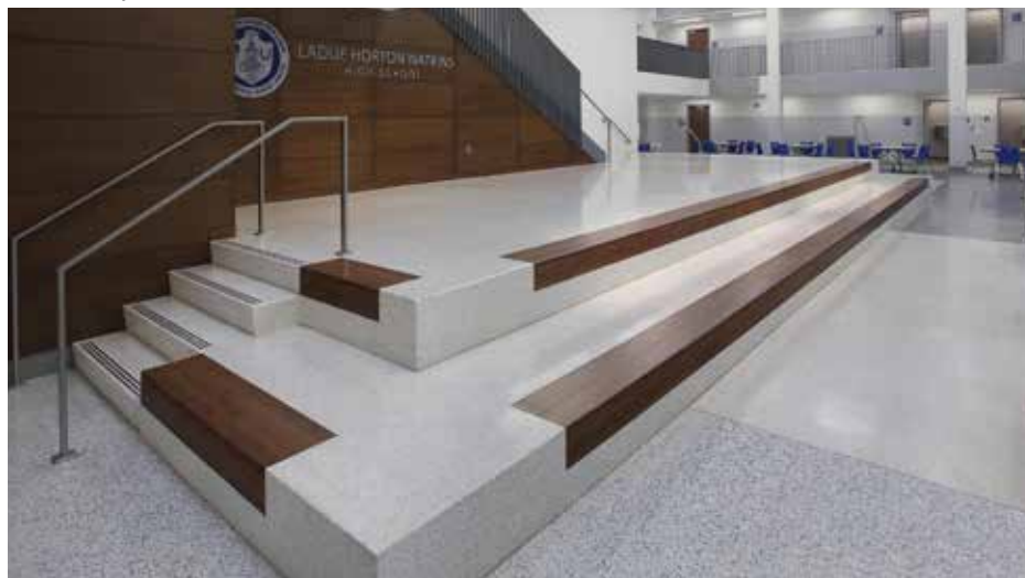
At Ladue Horton Watkins High School in Ladue, Mo., amphitheater-style seating with benches of poured-in-place terrazzo, inlaid maple seats, and precast terrazzo steps are featured in a new renovation and expansion.
