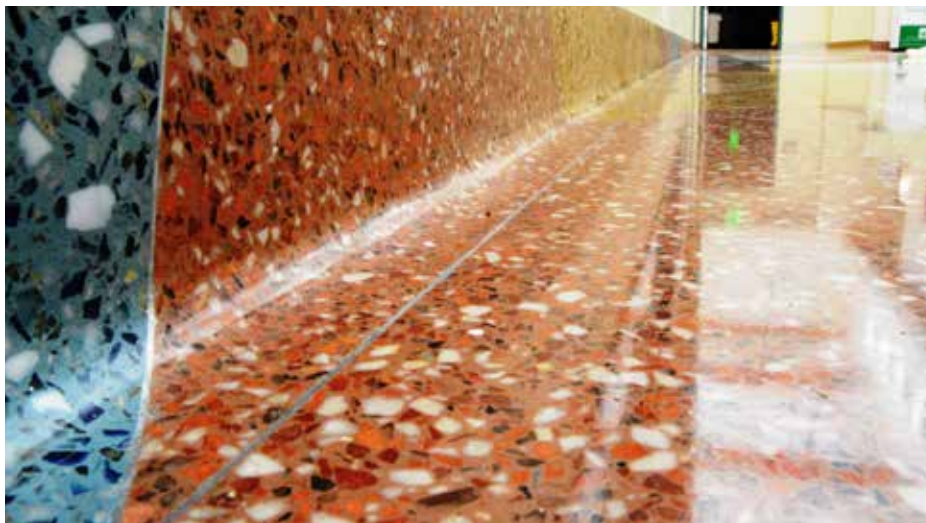
At the Pasadena Humane Society, terrazzo flooring seamlessly extends to the wall base.
