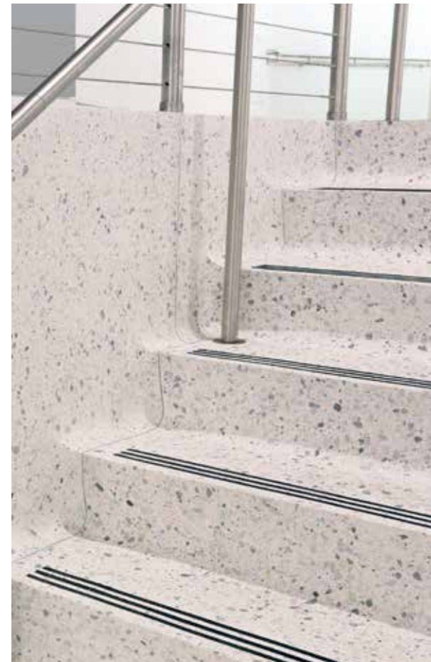
Venetian aggregate and a handcrafted, heavy-top divider strip create a clean, classic aesthetic for the floors, ramps, and stairs in the basement level of Houston’s Bank of America.
