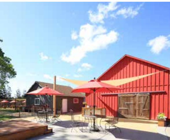
Redwood is a very sustainable material to use for outdoor spaces, such as the deck and posts shown here at a California winery.
