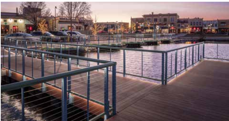
Cable rail systems combine posts and rails with stainless steel cables that minimize the obstruction of views and are made from sustainable materials.
