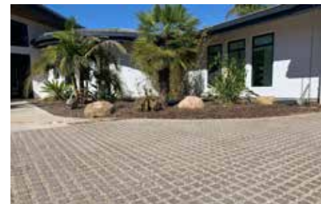
Flexible, permeable pavement systems can be used with a variety of infill materials including pre-cut artificial turf (shown on left), gravel, (shown on right), or vegetation, thus allowing for unique looks and applications.
