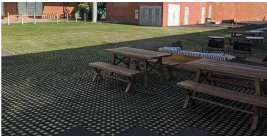
This Los Angeles project uses a flexible, plantable concrete pavement system for an exterior patio and vehicular driveway. Dolan Daggett, project director with Eric Owen Moss Architects, states “the beauty and performance of the product speaks for itself.”
