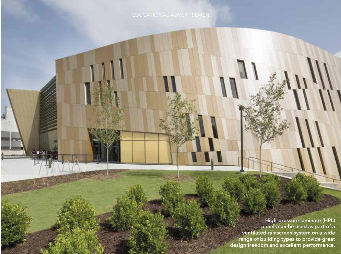
High-pressure laminate (HPL) panels can be used as part of a ventilated rainscreen system on a wide range of building types to provide great design freedom and excellent performance.
