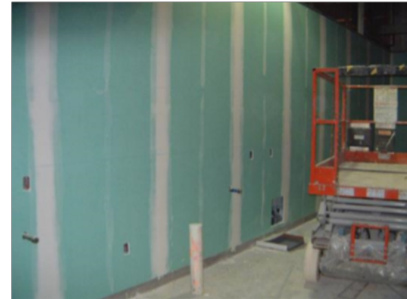
Example of Level 3 Finish
