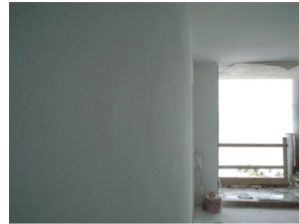
Example of Level 5 Finish
