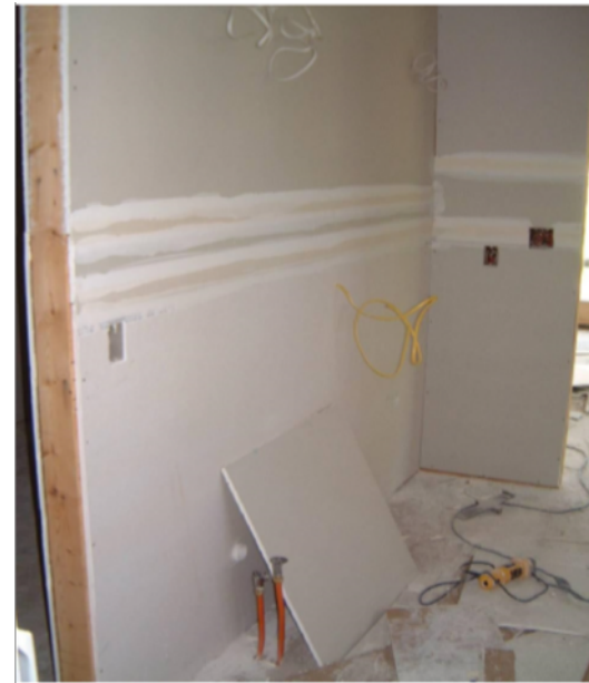
Example of Level 2 Finish
