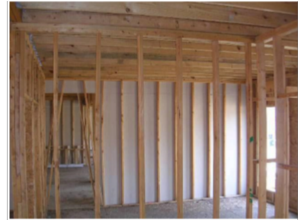
Example of Level 0 Finish
