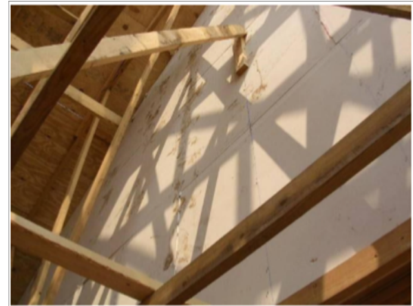
Example of Level 1 Finish
