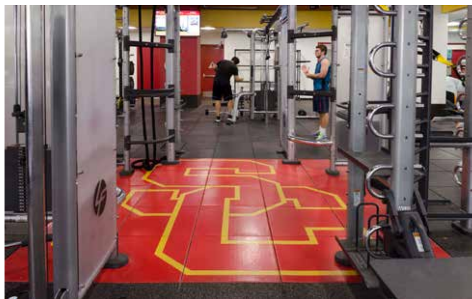
With student housing above, the University of Southern California's new Village Fitness Center needed to provide sound control at the source with performance flooring.
