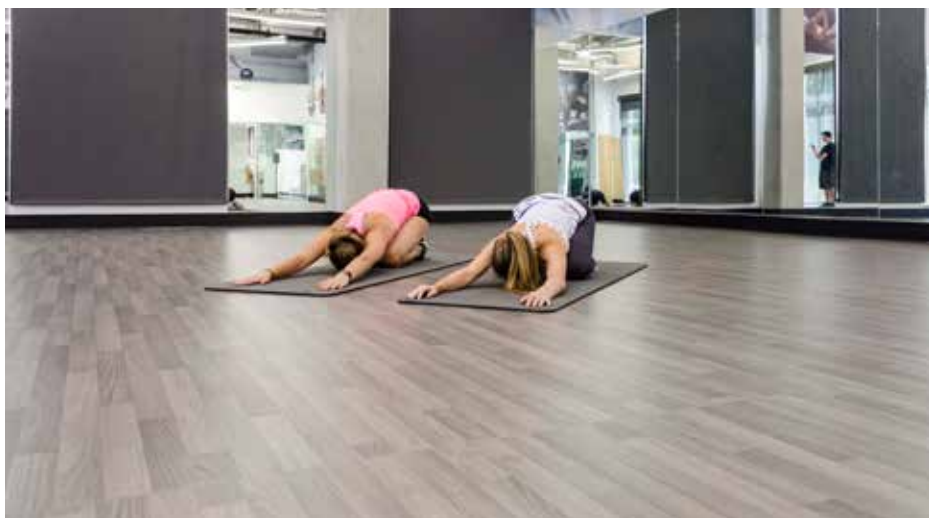
The design team selected an engineered performance flooring product that is 14.5 millimeters thick, combining a 2.5-millimeter wear layer with a 12-millimeter shock-absorbing base layer.
