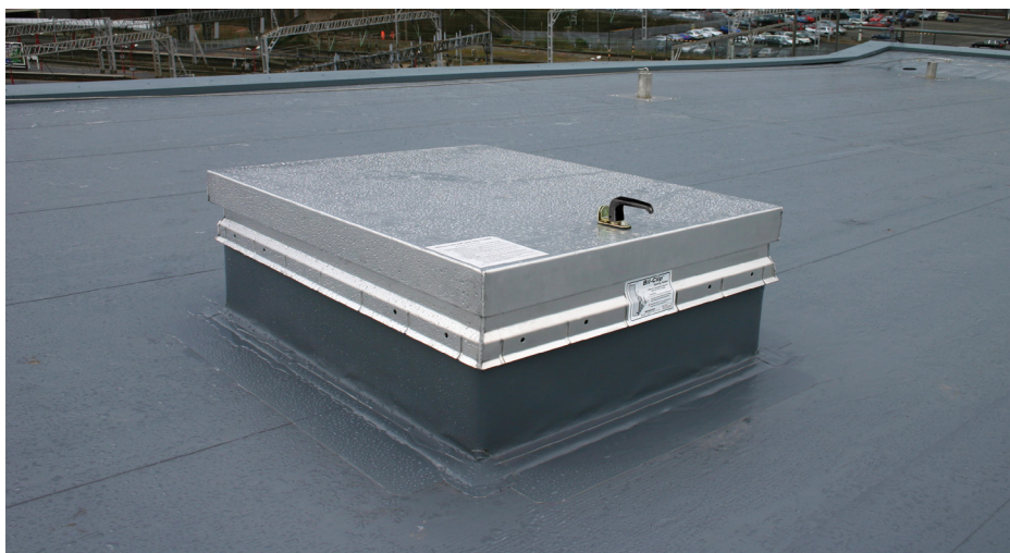
A thermally broken roof hatch.
