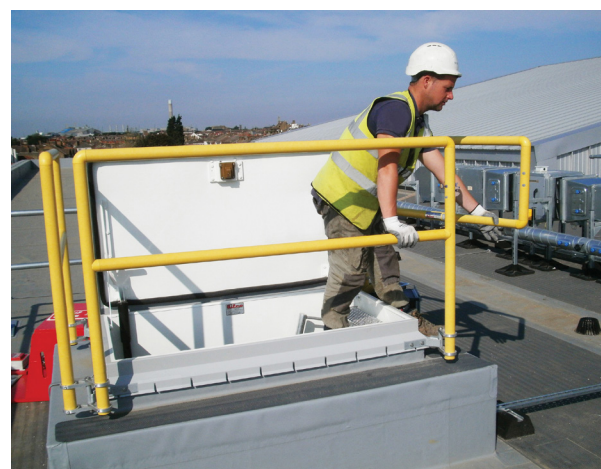
Fall protection is the main function of a roof hatch safety railing system.
